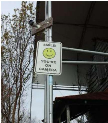
**SECURITY SYSTEM:** Shortly after the canopy was installed over the top of the house, a security system was installed. It has six independent cameras that provide 24-hour surveillance live and recorded. This system will be upgraded when the house is more stabilized to include inside motion detectors and possibly more cameras either hard wired or wireless.
