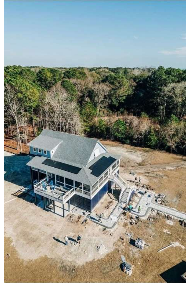
Aerial view — panels visible on porch roof
