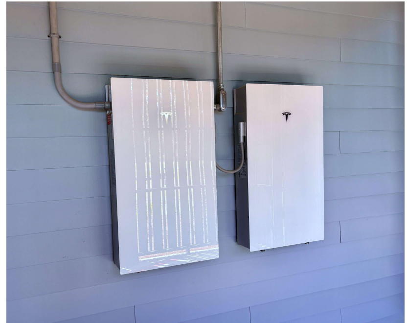
Powerwall 3 (left, with integrated inverter) and Powerwall Expansion (right)
